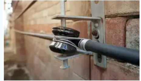
Spool insulator on Wall
